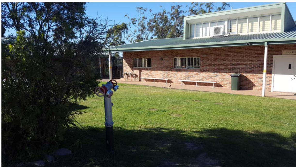
Photograph 6: Example of hydrant within centre grounds
